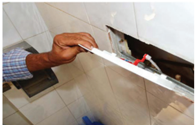
4. Clip the rod onto the new slim entry cover
