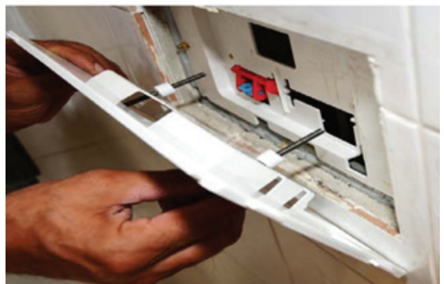
6. Screw the slim frame + the spacers onto the entry cover
