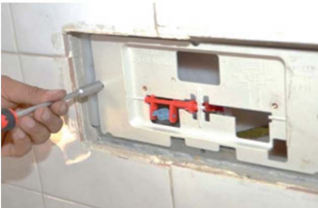
5. Screw on the new entry cover
