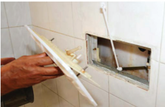
3. Unclip the rod from the entry cover
