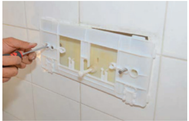
2. Unscrew and remove the support frame
