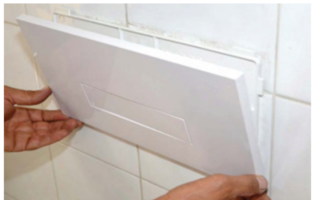
8. Engage the face plate from bottom to top
